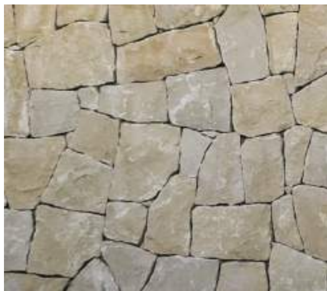
Cladding in outdoor areas. NATURAL DRY STONE MASONRY
